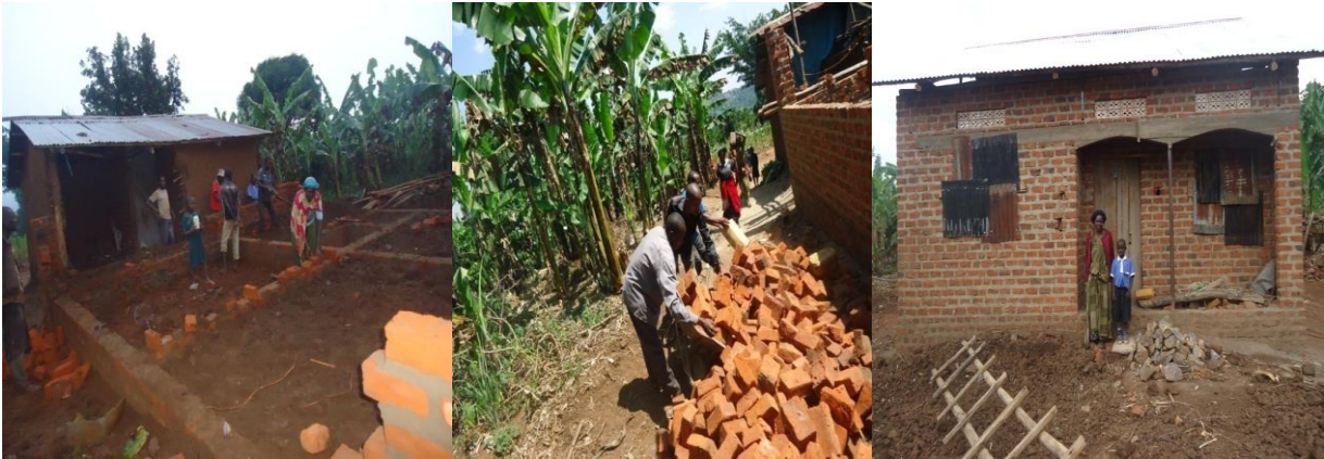
KAP members actively participating in the rebuilding of Rose's house
