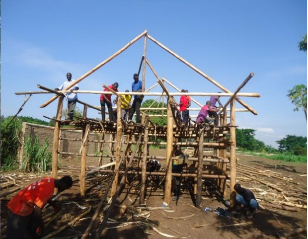
Students participating in the construction &
